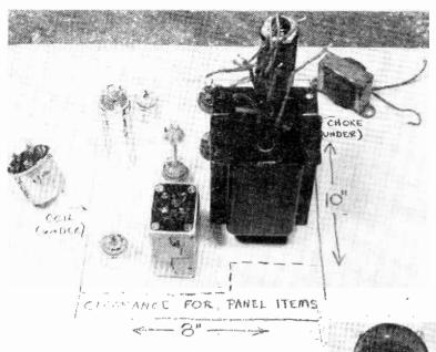
After securing all necessary components, lay out large parts on paper on flat surface and plan chassis layout. Photo below shows back of panel of corpleted unit.
