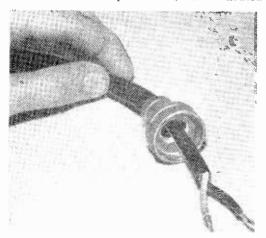
inside lengths of plastic garden hose. Bury the wire and hose, then caulk the open ends shut to prevent moisture from entering.—JOHN A. COM-STOCK.
