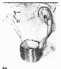
Wound coil ready for taping and varnishing. Start and 247th turn comes out left side and 257 to 292nd turns come out right.
