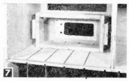
Skeleton structures are sufficient to support components, in this case, tuner and pre-amp.
