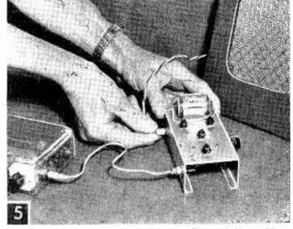
Connections between the radio and the amplifier and the amplifier and the speaker are made with plug-in cables. Shielded cable is used between radio and amplifier to avoid hum and other disturbances.
