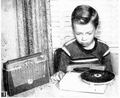
The Mini-player operates equally well in conjunction with a battery portable set as shown here, or with transistor, auto or line powered sets. Trim. three-speed motor is completely solf-contained.
