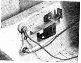
case, the current is led directly into the coil and the vibrating system is cut out. When current flows through the coil, the armature will be pulled down and thus release the bolt.—R. F. Y.
