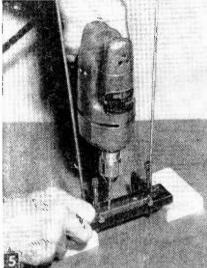
Drilling holes for 6-32 screws which attach terminal strip to base piece. Note that ends of antenna arms are put in position to line up the parts.
